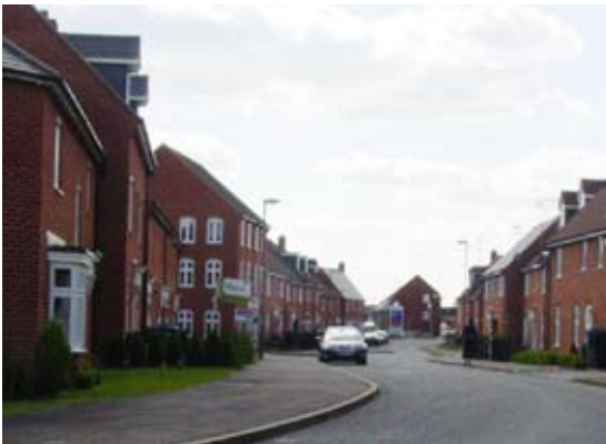
The Berryfields development in Aylesbury was admired for its coherent style and efficient layout.
