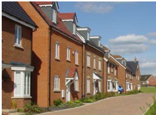
The recent Castlemead development at Pitstone (top and above) was cited as an example of a place with certain good qualities to aspire to.
