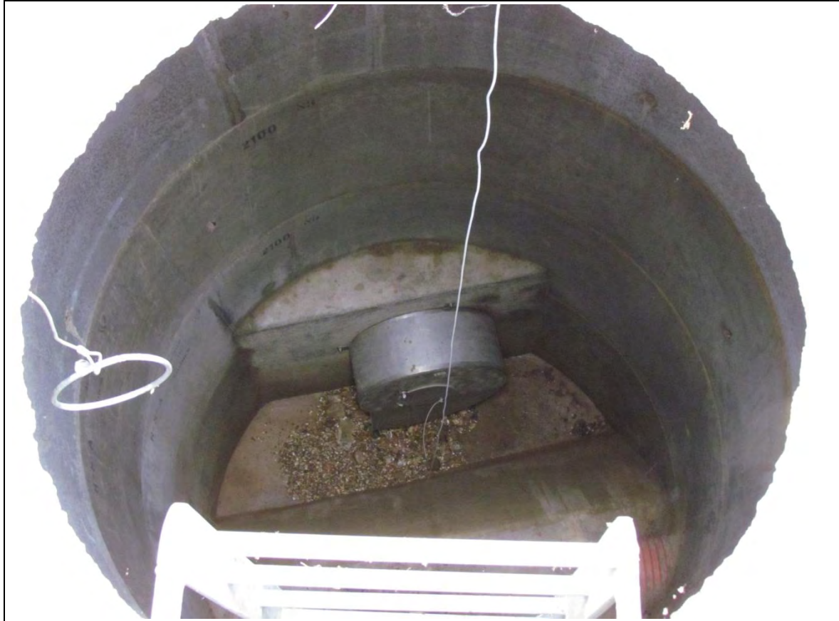
Figure 3.7 Flow control chamber adjacent to existing depression
