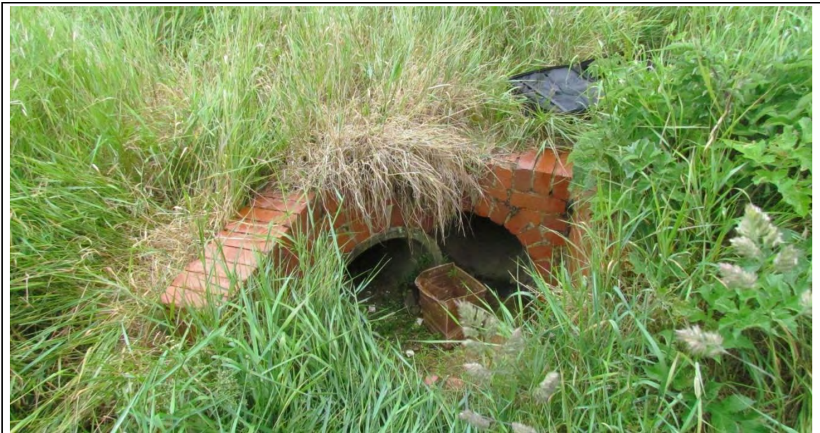
Figure 3.3 Headwall at the downstream end of the ditch
