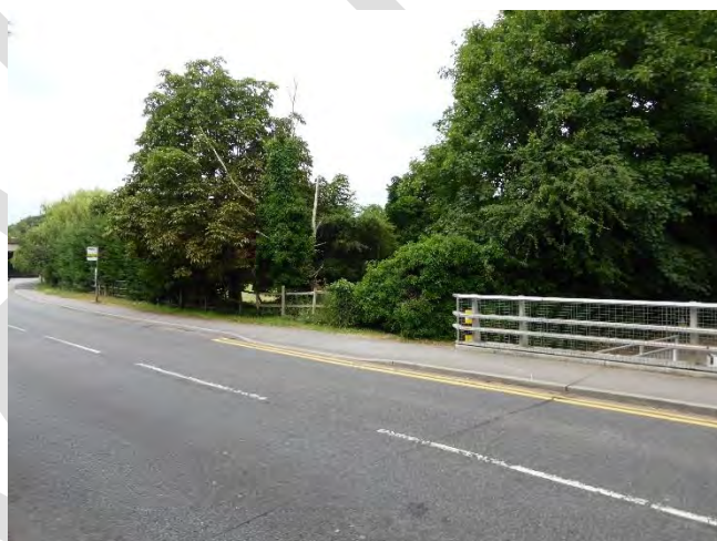
Figure 35 - Access, north side
