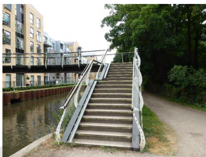
Figure 37 - View from north
