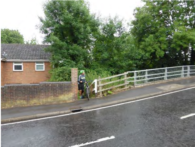
Figure 22 - Access on south side, east bank road end
