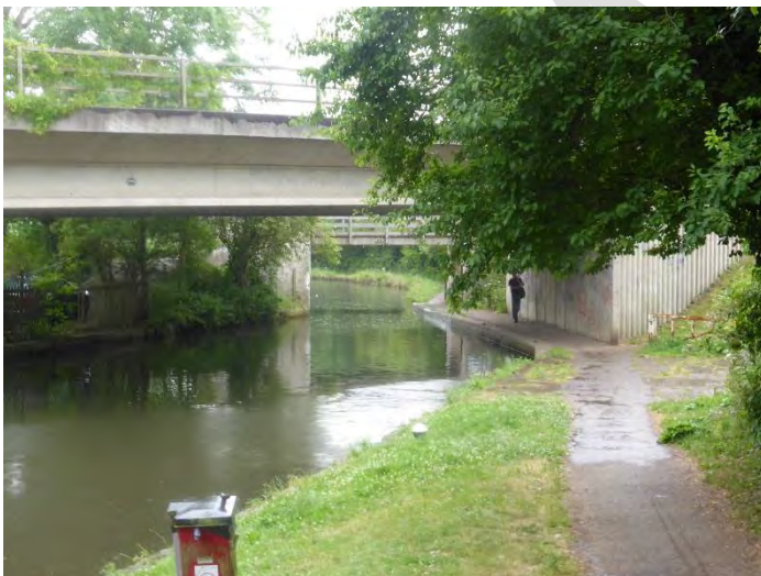
Figure 14 – View looking south
