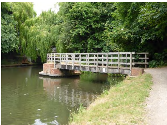
Figure 27 - View looking north
