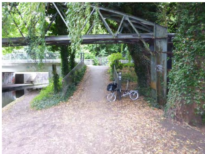
Figure 32 - Access to road, south side
