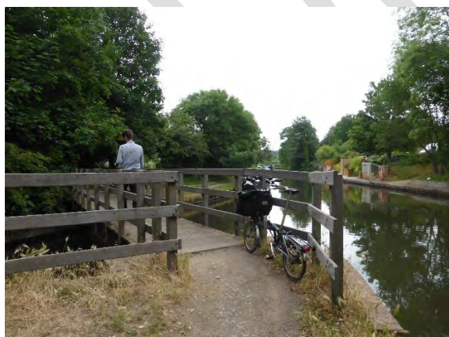
Figure 31 - Bridge looking south
