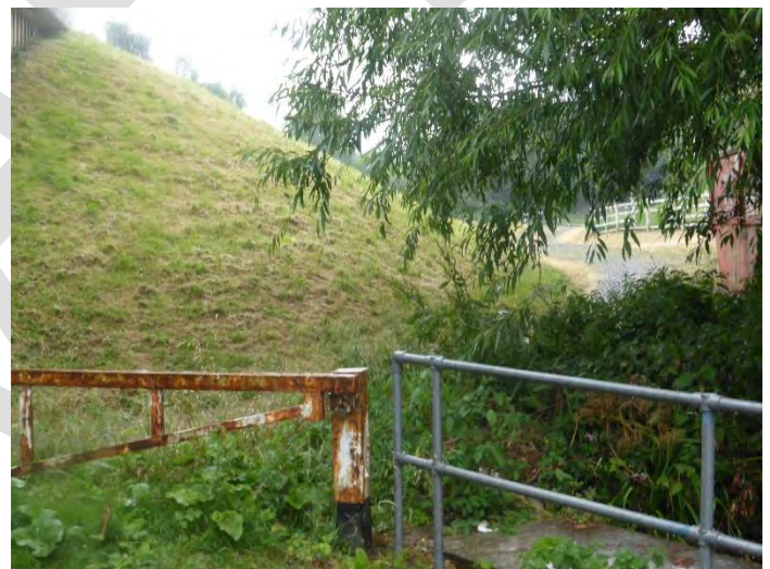
Figure 15 – Access on north side, west bank
