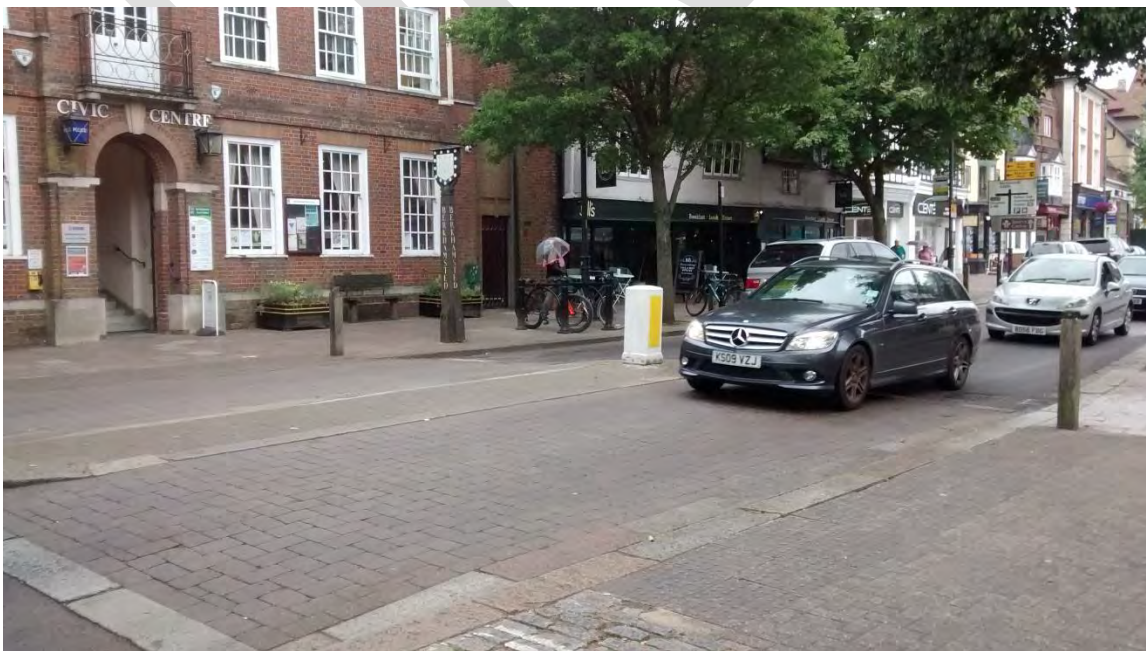
Figure 42 - Raised table courtesy crossing in Berkhamsted
