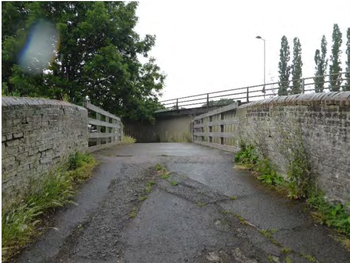
Figure 13 - Bridge deck looking west
