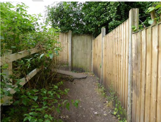
Figure 20 - Access on south side, east bank
