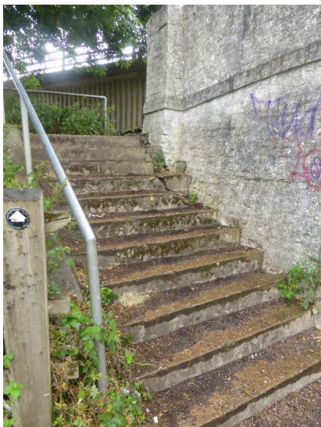
Figure 11 – Steps to towpath on south side, west bank
