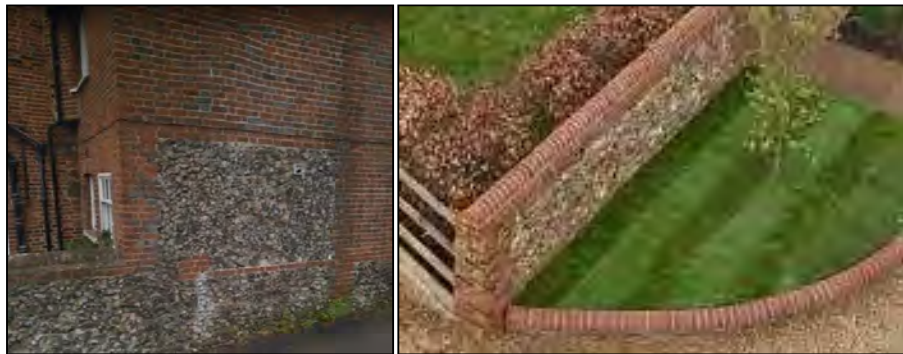
Use of flint at Langley Hill; Flint incorporated at Hill Farm redevelopment
