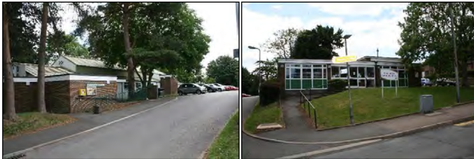
Images show: Kings Langley Community Hall and Kings Langley Library
