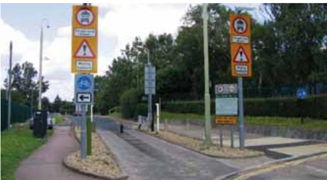
Rising bollards that give priority to buses
