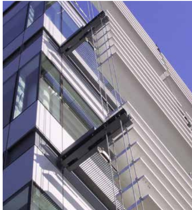
Horizontal louvres at 300 Longwater Avenue
