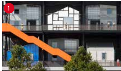
The 'Olympic' Park facing façade has a number of modular artist studios for the community to use.
