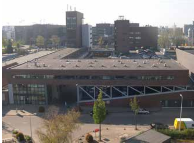
Example showing attractive frontage facing the public realm with concealed servicing yard located at the back
