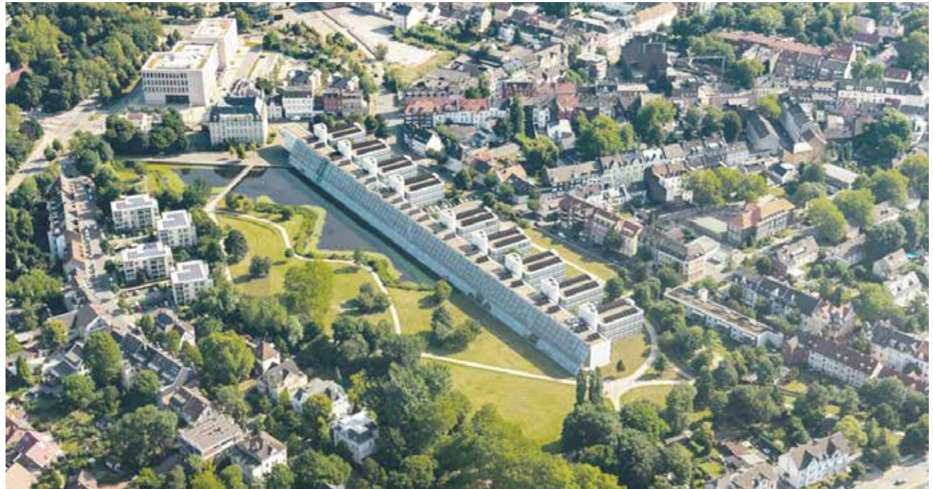
Tilted and interactive glass façade at the Gelsenkirchen Science Park, with PV Solar Plant on the Roof
