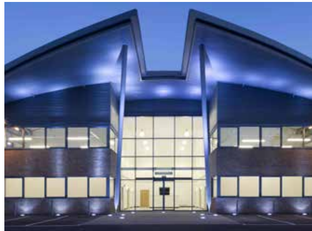
Entrance area with social hub area on the ground floor at Maylands Business Centre. Photo: DBC
