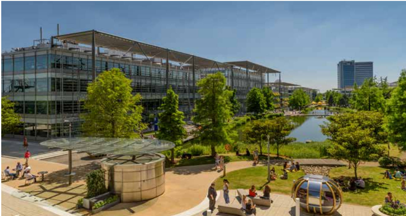
Solar shading at Chiswick Park
